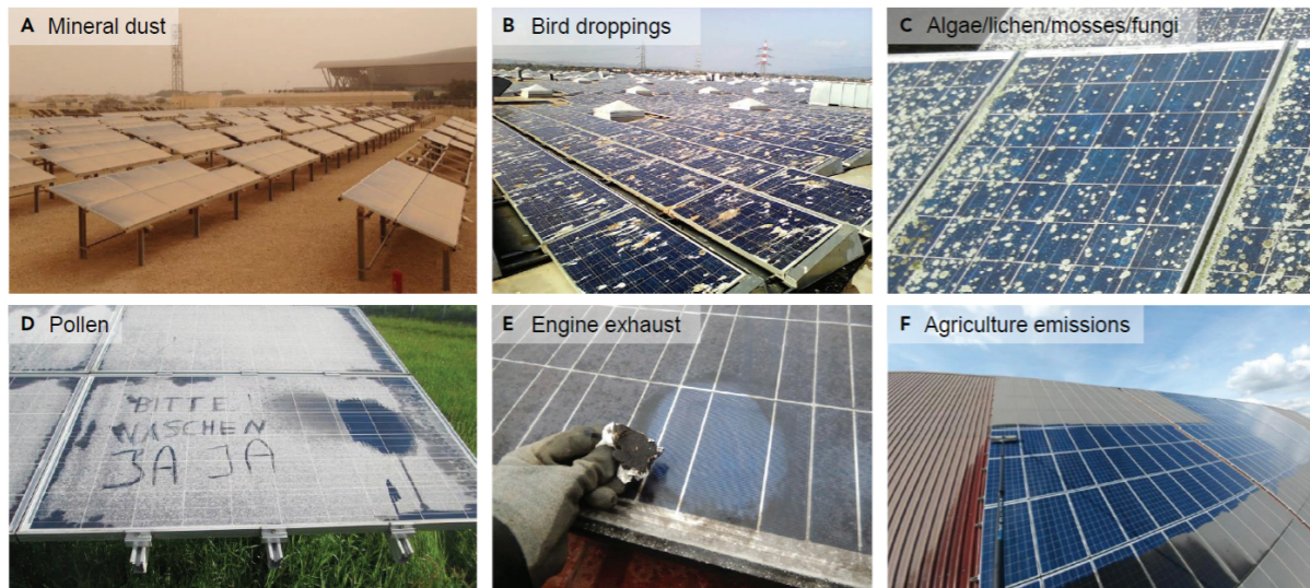
Figure 01: Examples of Soiling [1]
